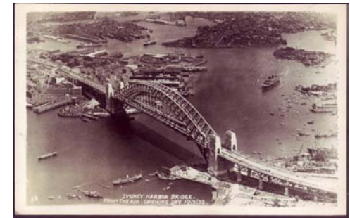
The Sydney Harbour Bridge was opened in 1932. The landmark linking Sydney's northern and southern shores began construction in 1924 and took 1,400 men eight years to build at a cost of 4.2million pounds and 53,000 tonnes of steel. A toll was established and during the first year the average annual daily traffic was around 11,000 vehicles, growing to around 160,000 at the beginning of the 21st century. The bridge is used on each New Years Eve for the grand finale of a spectacular fireworks display around the harbour. Card producer unknown, shows Kodak-Austral back.
