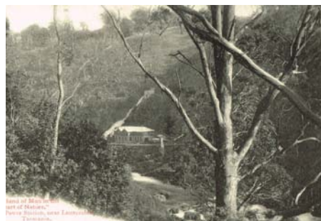
Electrical Power Station. Card produced by Richard Gee, Launceston.
