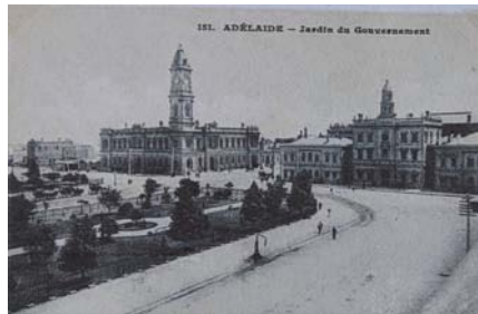
"Government Buildings" c 1880. G.P.O. and Treasury Buildings
