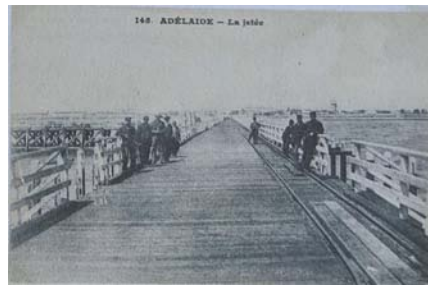
French seamen relaxing on the Semaphore Jetty in 1885. (note the rails at right for the hand truck)
