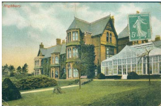
Highbury with glasshouses to the side.
